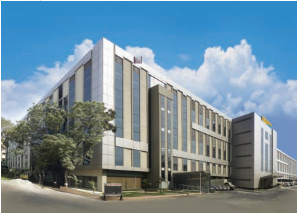
Switchgear Factory, Mumbai
